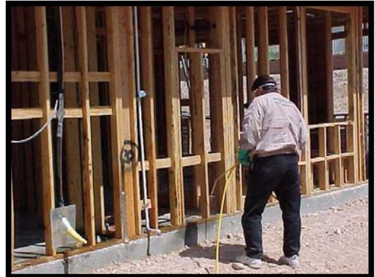
Borate based pesticides used in Nevada for the pre-treatment of wood upon slab type foundations is applied directly to wooden members, utility penetrations and in some cases concrete surfaces as specified by the pesticide label. The use dilution of these pesticides is applied as a liquid solution to all exposed wood surfaces "to a point of wetness" by sprayer, brush, or roller.
