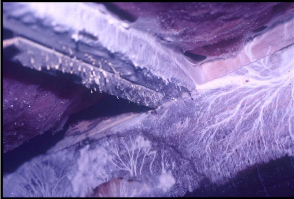
**“Active infestation” of Decay fungi on joists in crawlspace**
