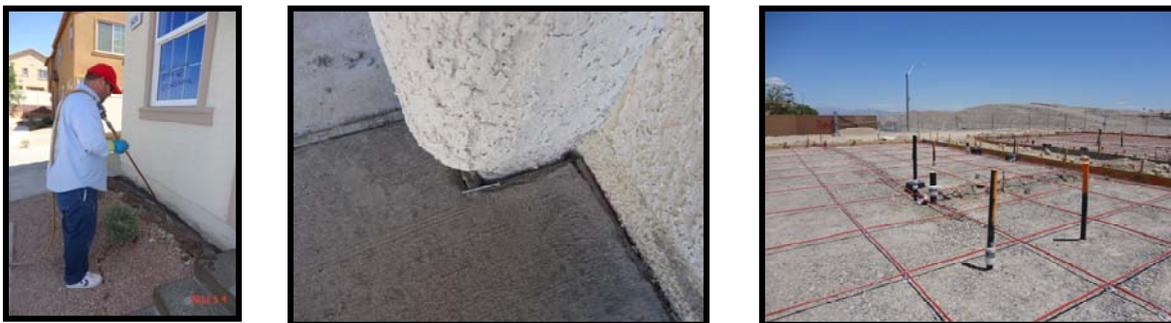
Effective termite control requires termiticides be applied as a continuous barrier in the soil next to and under the foundation. Establishment of vertical barriers adjacent to vertical surfaces includes treatment of the soil adjacent to the perimeter of the structure, cold joints where two slabs abut, and utility penetrations which protrude through cement slabs.
