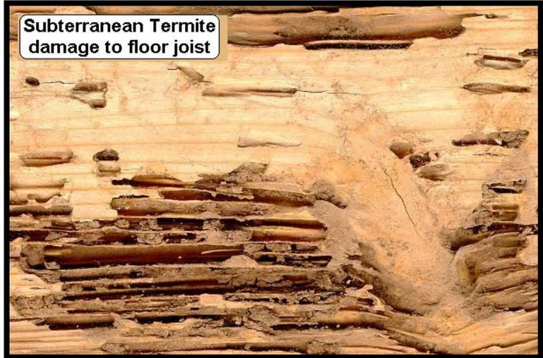
**Damage by Subterranean termites, notice area near the bottom that appears to have been etched.**
